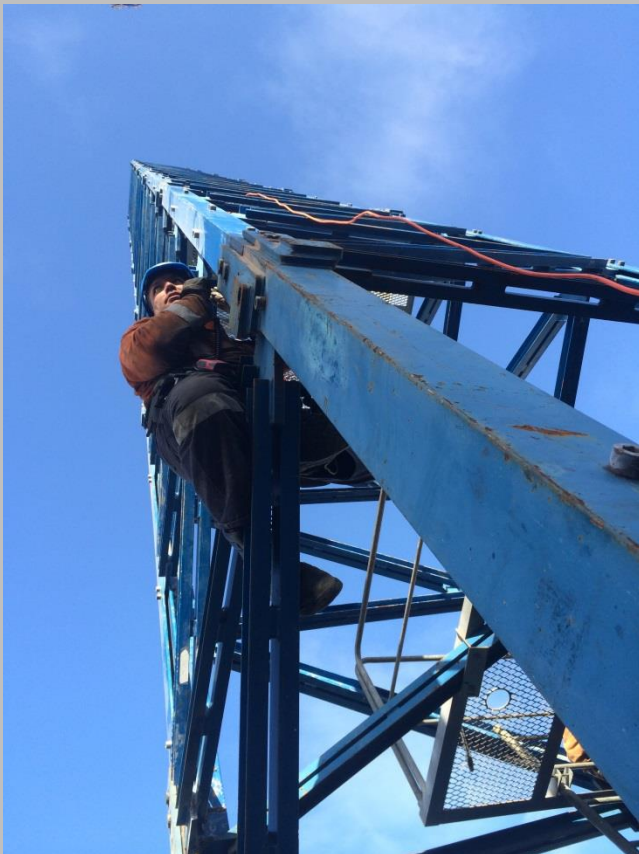
Erection and dismantling of clients tower cranes and hoists
