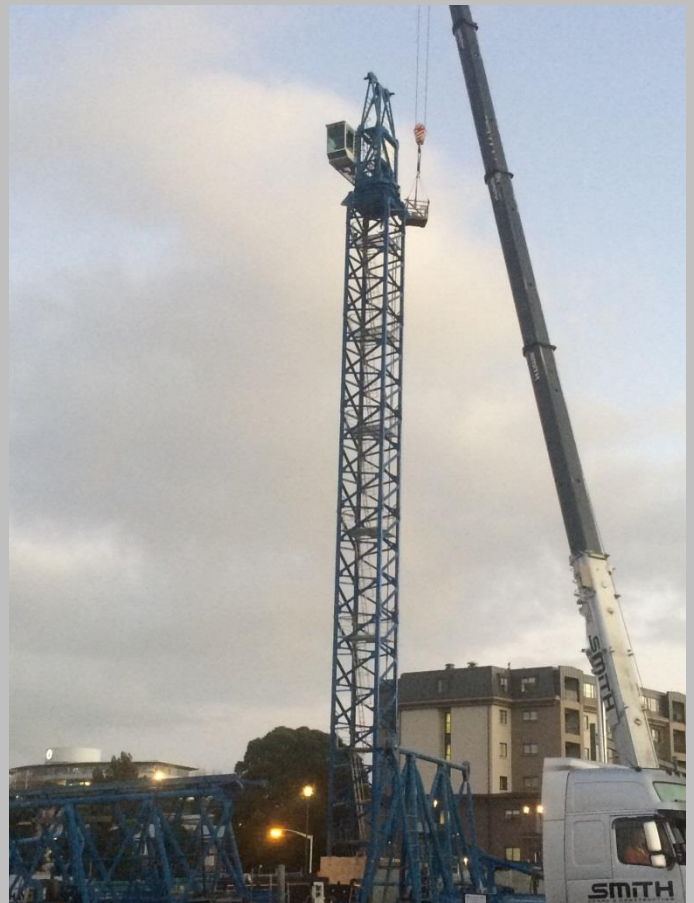
Erection and dismantling of clients tower cranes and hoists
